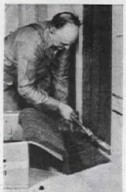
Kimsul blankets come in widths which exactly fit between standard studding—save cutting and measuring on the job.
