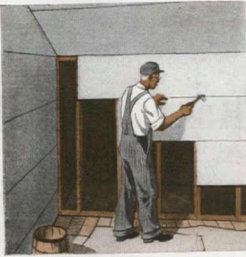
1 and 2. Rigid insulating board
