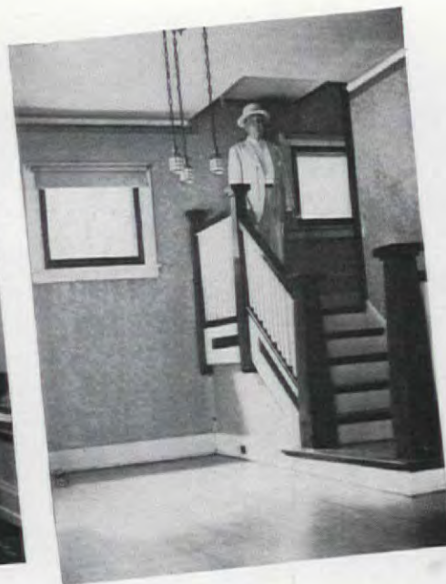
The stairway was turned so as not to waste wall space. The ugly square window was exchanged for a full sized one. The dreary center fixture was removed
