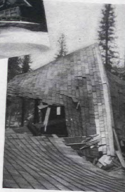
Heavy snowfalls in the California High Sierras demolished this bad roof construction
