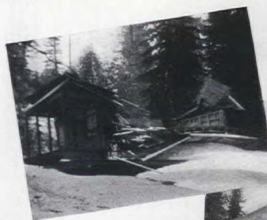
Heavy snowfalls in the California High Sierras demolished this bad roof construction
