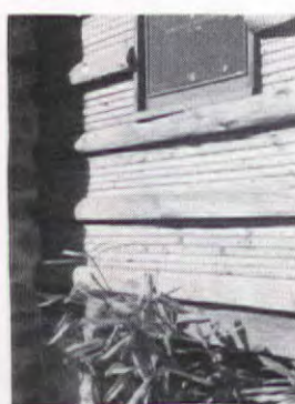
Wood board or block cabin construction. Half logs at intervals vary exterior treatment
