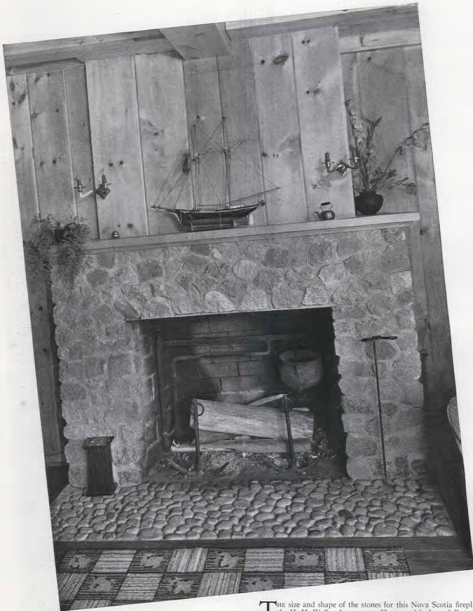
Cobblestones picked up on the beach are used for the hearth; adjoining walls, covered with light knotty pine board, have concealed closets
