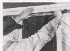
Attached to top plate with lath and nails...
