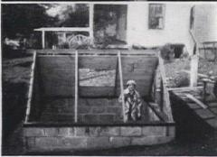
The north side of the roof was boarded up except for the central window space, as shown here. The south side consists of three standard 5 by 6 ft. hotbed sash (see above, right). The door, steps, and one ventilator are at the east end
