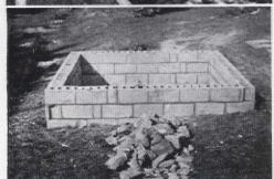
Then professional labor leveled the floor, poured the footings and laid the hollow tile foundation—all in one day. On this we bolted sills and erected rafters for an even-span roof as shown below. . .
