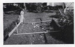
Nothing difficult or expensive about building this greenhouse. First, we staked out and dug the 9 ft. 4 in. by 8 ft. 10 in. excavation—three feet deep it was...
