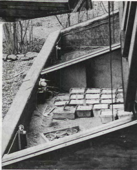
Almost human in its operation. Thermostats control the furnace-damper motors (on garage wall), which raise and lower the sash
