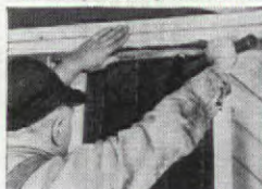
Attached to top plate with lath and nails...
