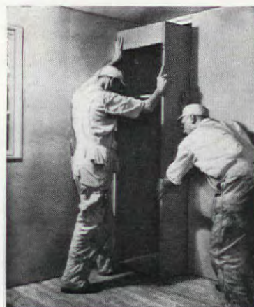
Putting a ready-made fire-proof steel closet in place
