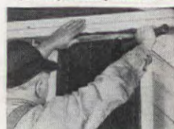
Attached to top plate with lath and a few nails.
