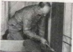
Nailed at bottom and cut off —that's all! Strong rows of stitching keep KIMSUL perma- nently in place.
