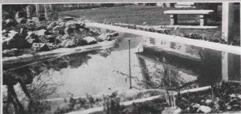
At last it was finished—glistening white and waterproof beyond a doubt. Note one fountain standpipe and the plant “shelves” on the far wall. During the impatient days of washing and filling, the margins were planned and planted
