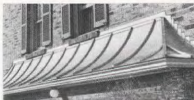
This graceful batten-type canopy roof offers ample evidence of the excellent shaping qualities of ARMCO Stainless Steel.
