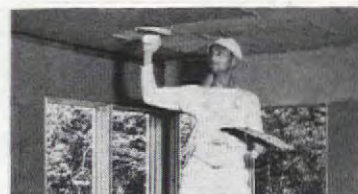
Better Plastering Base. Fir-Tex Insulating Board Lath is the modern and economical way to prepare walls for plaster. This solid base prevents lath marks . . . plaster cracks are minimized.
