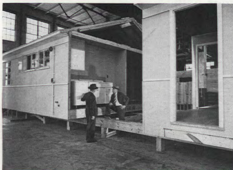
Portable houses, built in sections in factory, have wood framework, insulating board walls in and out
