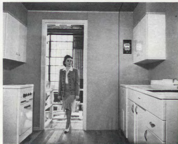
Plumbing and wiring are put in at factory, including fixtures; all plumbing is in single section
