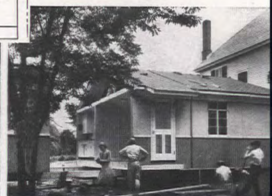
Sections are reassembled on site
