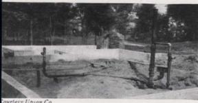
Foundations go 4' below grade line, plumbing lines are installed before 4" concrete slab floor
