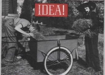
It hauls everything from dirt to dishes in its roomy box. Made of pine, it rests on individual suspended axles. Half-inch water pipe makes the one-piece handle. The end of the cart, held by screen hooks, can be opened for dumping. NETTIE MAE DEFFNER, Parkville, Mo.
