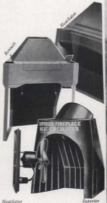
Don't forget that your fireplace will be a cheerless thing if it doesn't work satisfactorily, no matter how charming it looks. The parts of a fireplace must be properly proportioned and necessary equipment installed. Fortunately, definite standards of fireplace design are established now and modern equipment is reliable. Especially helpful are these ready-made units providing the basic skeleton of the
