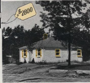
new methods the designer, Mr. Howard Fiedler, used in building the houses and expediting their construction; no cellars, concrete slab foundations, speedy plumbing installation, interior and exterior walls erected independently of each other, wall finishes for rooms in single panels, co-ordinating of all construction work so that a house goes up like clock-work and can be enclosed in four days. Even in these days, that's speed!
