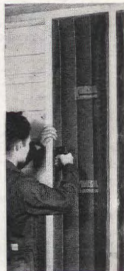
Picture shows KIMSUL blanket being installed in side wall of a home. Note the neat, snug-fitting insulation job which one man can do quickly and easily with KIMSUL.
