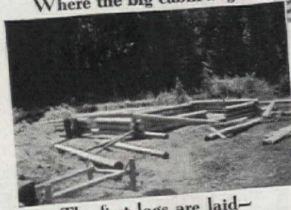
The first logs are laid—
