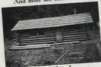
Until the roof is done—
