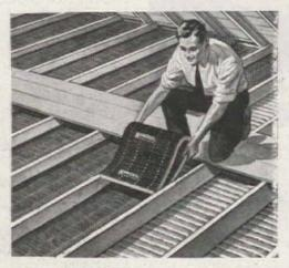
FITS LIKE A GLOVE-KIMSUL fits snugly between the joists in your unfloored attic. Simply fasten one end of the blanket at junction of floor and eave. Stretch it taut and fasten to opposite eave. Repeat for each open section of the floor. That's all! If your attic is floored, apply KIMSUL between the rafters of your sloping roof.
