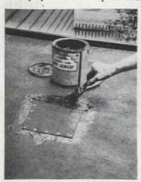
Patch has been nailed to hole in old tin roof. A heavy coating of roofing cement is then applied over patch and adjacent roof
