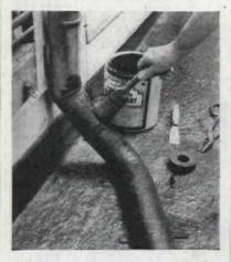
Defective joint in leader connection is filled with caulking and then painted with heavy coating of roofing cement for protection
