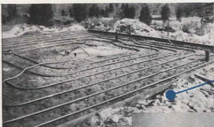
Coiled heating pipes in concrete slab under parquet floors and between ceiling joists
