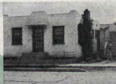
A cracker-box house was rejuvenated by adding a Monterey farmhouse-type porch
