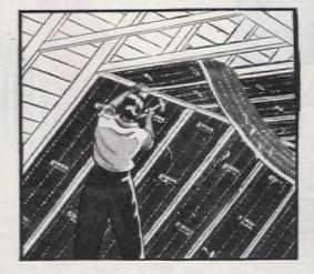
Fits Like a Glove-The KIMSUL blanket effectively insulates your home because it fits snugly between joists of the unfloored attic . . . or between rafters of the sloping roof, if your attic is floored. Anyone who can use a hammer can install KIMSUL. What's more, it is pleasant to handle-contains no harsh, irritating ingredients.
