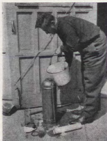
Dissolve soda powder, pour into shell, and add water until full
