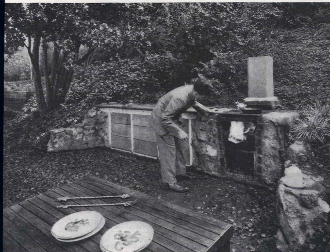
A barbecue unit of gray field stone cut into steep garden bank was Frazer M. Cole's idea. Cupboards for storing coal and wood—with top usable as chef's table—are painted gray; chimney is made of yellow plaster
