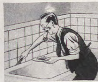
FIX CRACKS IN TILE, WALLBOARD
