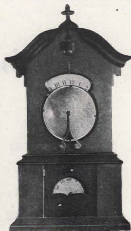
Terrestrial clock: globe revolves every 24 hours, dials indicate hours and minutes. Designed and made by Timby, an upper New York state clockmaker
