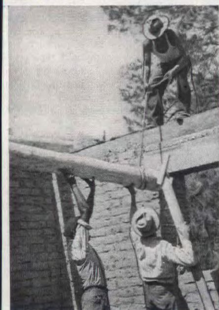
Pine poles being lifted into right place to form the ceiling rafters
