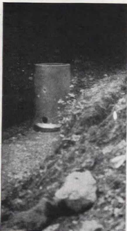
This is the drain water tile tank in place 13 ft. below the spring where it bubbled up out of the hillside
