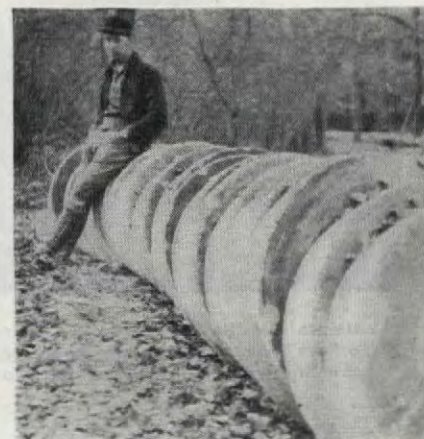
The 40 castoff grindstones (400 lbs. and 35 cents each) which made the dam that the Bardsleys built
