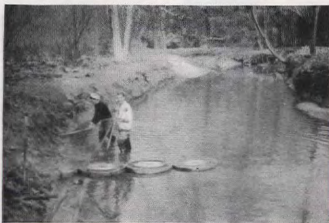
The heavy grindstones were rolled and pried into place with long bars made of small trees. This shows one tier in place and a start being made on the second
