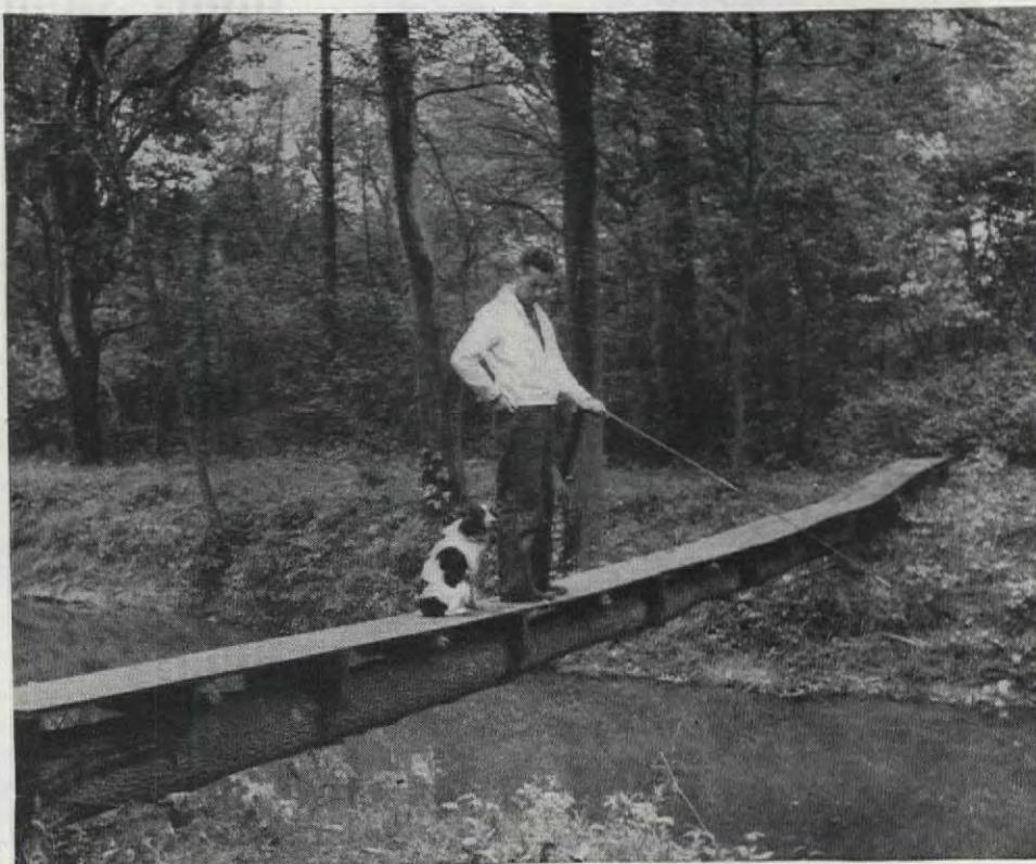
The present foot bridge across the 30 ft. creek, built of cross pieces and planks supported by a single tree, is adequate but temporary. Some day it will give way to a more commodious (if less exciting) rustic bridge, says Dr. Bardsløy
