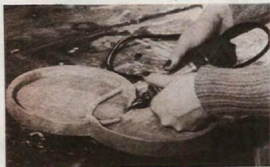
A twin tray is achieved from a single piece of wood, with band, jig or coping saw and router
