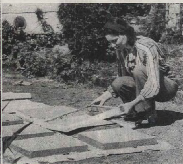
4. And deftly removed the wooden forms when the cement had fully hardened
