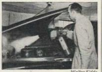
Always ready in the garage is the extinguisher which will put out the fire and leave the car engine intact
