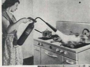
and effective Simple is this small carbo extinguishe for the fat fire or working surface kitchen range
