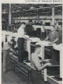
Installing the glass wool insulation on electric ranges; it is also used in better gas ranges
