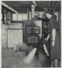
Nipped in the bud is this fire at the oil burner, for the simple carbon dioxide extinguisher was handy
