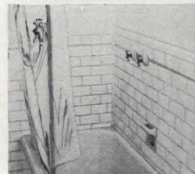
Step 4. The finished product; gaping holes are gone, tile is firmly fixed. The operation consumes about two or three minutes per tile—no fuss
