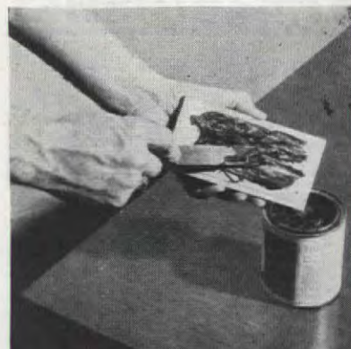
Photograph shows how a different type of compound is used. Material is "buttered" on tile with an old kitchen knife—it's sticky, though, so don't get any of it on your hands
