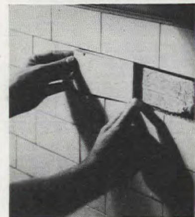
Step 3. The tile is put in place, pushed firmly against backing material
