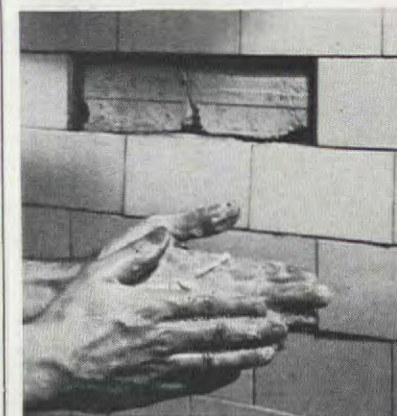
Step 4. The finished product; gaping holes are gone, tile is firmly fixed. The operation consumes about two or three minutes per tile—no fuss
