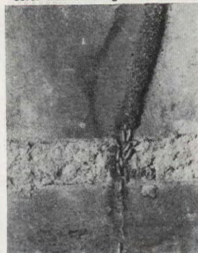
Broken tube reveals workers going to and from colony. Termites die on exposure to light and air
