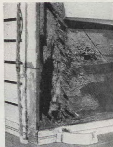
Damage to wood siding. Partly excavated or unexcavated soil area beneath ground floor is danger spot
