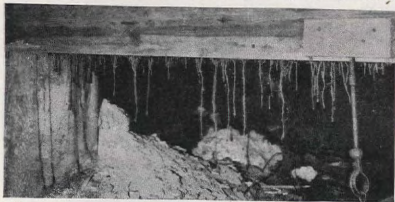
Moisture is essential to termite life. Stalagmitelike tunnels connect underground termite colony in earth with structural members of house
