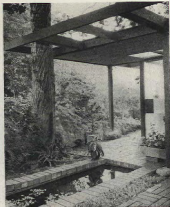
Lily pool near entrance, plus louvered screen, stop callers from stepping back onto main terrace. This affords greater privacy for owner and guests . . . roof trellis, ingeniously built around tree, was used to preserve natural planting
