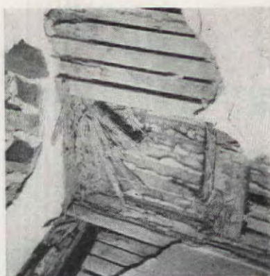
Termite damage to this interior wall was discovered only after outer wall covering was removed
