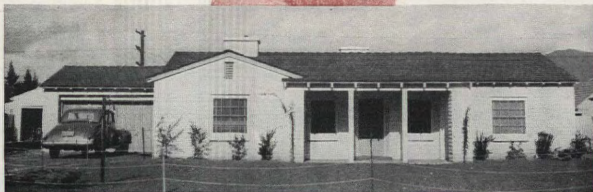
A stabilized earth house can be built anywhere if proper proportions of sand and clay are present in soil
