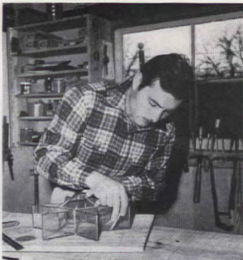
An amateur when he started his home, Montgomery is an expert cabinetmaker now. At left and below, some steps in mounting the fine antique lamp fixture with pine backing, copper frame and glass panels shown at right
