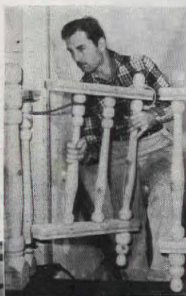
George mounts a section of the railing which he turned, made, and finished in his work shop
