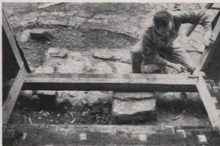
Next step is to cut hole in wall for fireplace. Second hole, in floor, is for hearth. Here, cut floor joists are being braced
