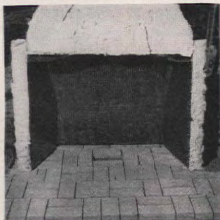
Brick nears top of circulating unit. Soon step backs will be made, as fireplace ends and chimney begins. Some bricks protrude to provide rustic effect. Clean-out door, referred to on page 69, may be seen standing ajar at bottom
