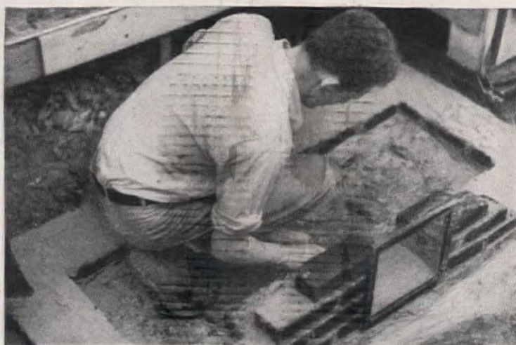
Next step is to cut hole in wall for fireplace. Second hole, in floor, is for hearth. Here, cut floor joists are being braced
