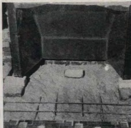
Bill is joined by his wife, Dorothy, in laying brick up and around heat circulator. Here they are beginning to work on the tenth brick course. Bricks are laid in double rows for the side walls, while only a single row is necessary for the rear wall.
