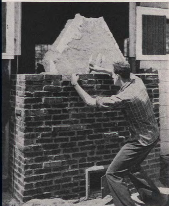
Brick nears top of circulating unit. Soon step backs will be made, as fireplace ends and chimney begins. Some bricks protrude to provide rustic effect. Clean-out door, referred to on page 69, may be seen standing ajar at bottom
