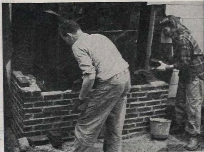
Bill is joined by his wife, Dorothy, in laying brick up and around heat circulator. Here they are beginning to work on the tenth brick course. Bricks are laid in double rows for the side walls, while only a single row is necessary for the rear wall.
