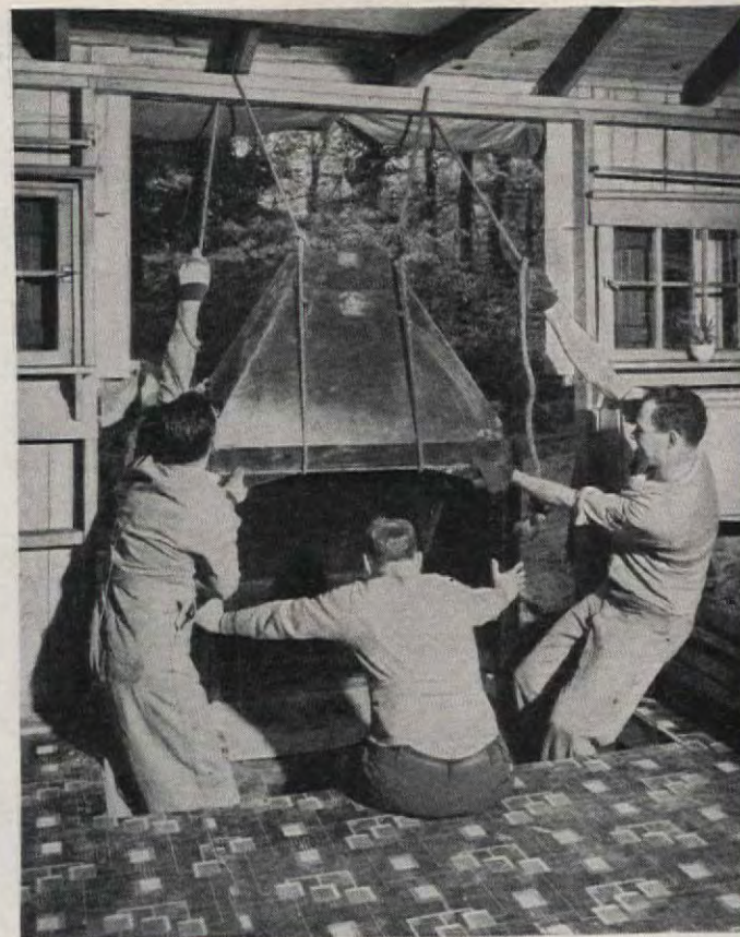
Fireplace walls have now reached the height of the room floor. Here Bill, Bob, and another friend are installing the heat circulator unit for the fireplace. If boys had not had the beam handy, unit could have been moved on blocks and rollers
