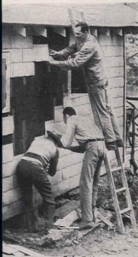
Plans call for fireplace to be located between two side windows. First step is to remove shingles from that area
