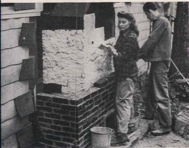
An important step for safety is installation of rock-wool insulation on circulating unit. Here Dorothy is joined by friend, Bob, at this task. A mixture of Portland cement and water, to the consistency of paste, was used as an adhesive
