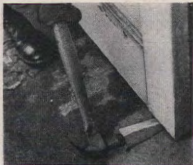
Wedge is driven under the door to square it before the plywood stiffener or wood brace is installed
