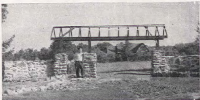
Roof frame is in place, supported on 4 x 4's set down on pipes and creosoted. Note proportions and pitch of roof
