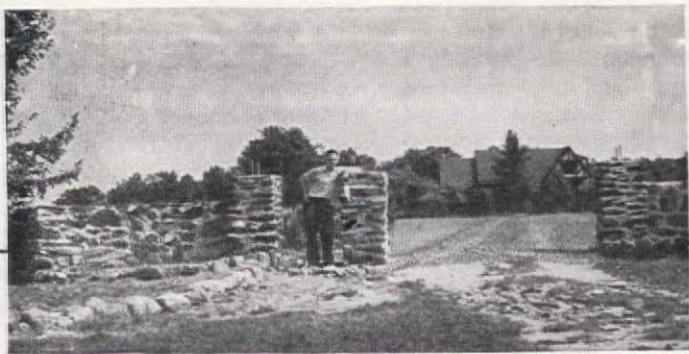
An early stage, with fieldstone walls and posts finished. Note the two projecting anchor pipes at top of each post
