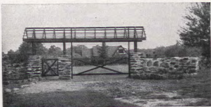
Frame is now complete with horizontal supporting slats, ready for the belfry frame—and the actual thatching
