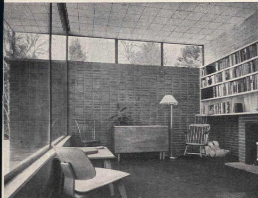
● Throughout the house the juxtaposition of heavy masonry and light framing was used for wind bracing and esthetic contrast. Red-birch plywood thus vies for focal interest in living room with modular brick wall pattern, and the insulating glass of sash
