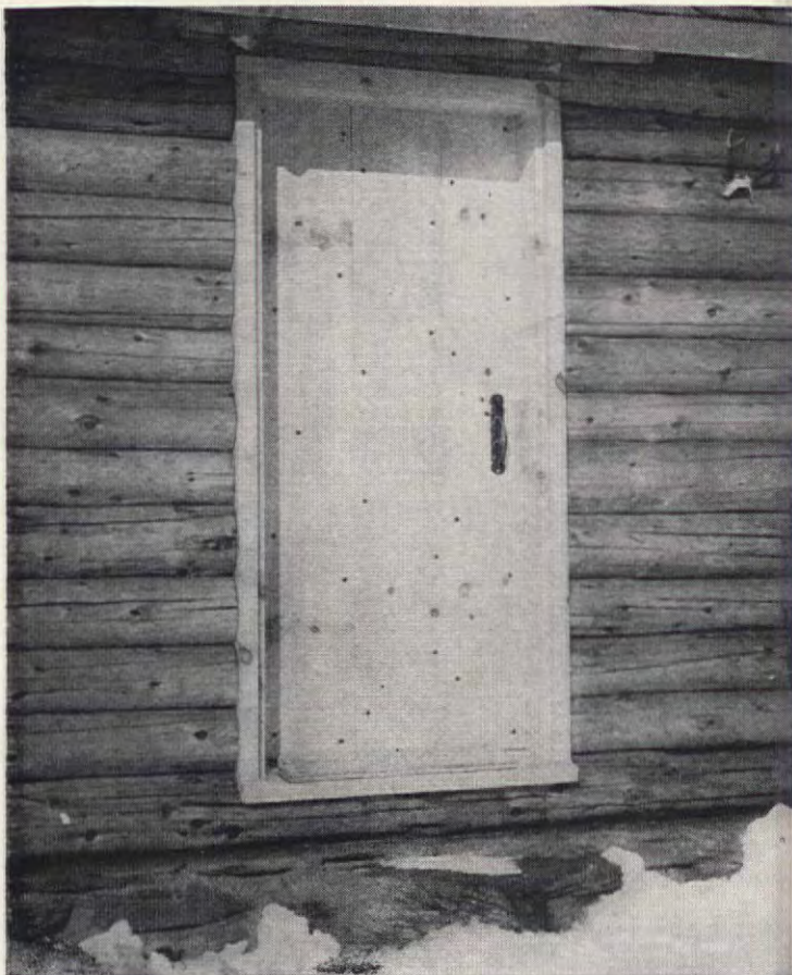
Door is made of two layers of white pine boards with one layer of spruce between, lag screwed firmly together
