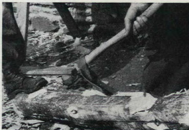
With a "shin-hoe," or howel, the marked log is hewn to a tight, neat fit that sheds water
