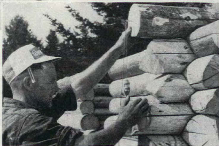
The rough-notched log is laid in place and lined up plumb before marking for the finished cut
