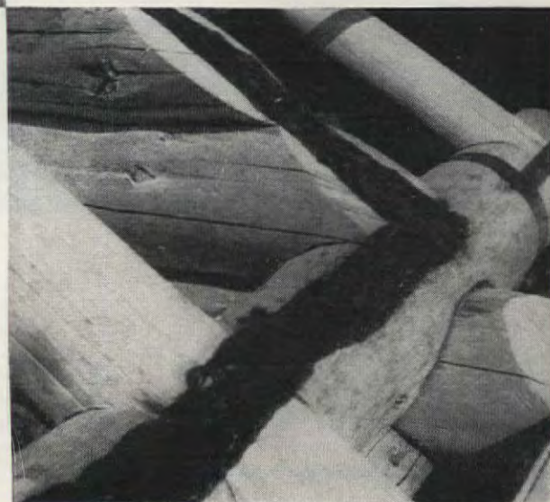
Plate and gable-end logs are strung with oakum to insure a tight fit when ceiling boards are nailed in place. Notice the tight fit where the rafter and plate logs meet
