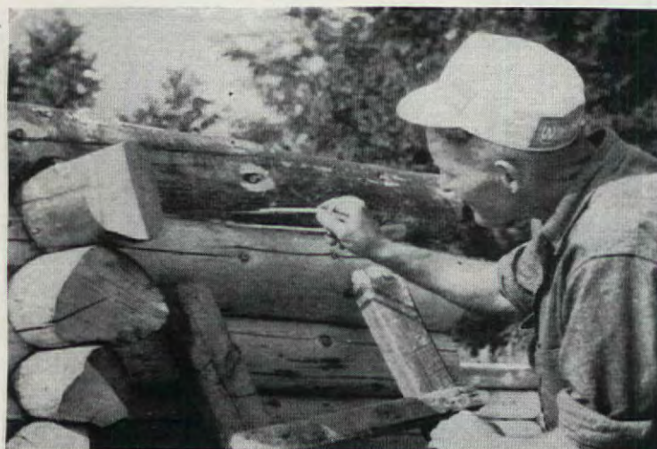
Crayon is used for marking the log after it is lined up. Pencil is useless on the smooth surface
