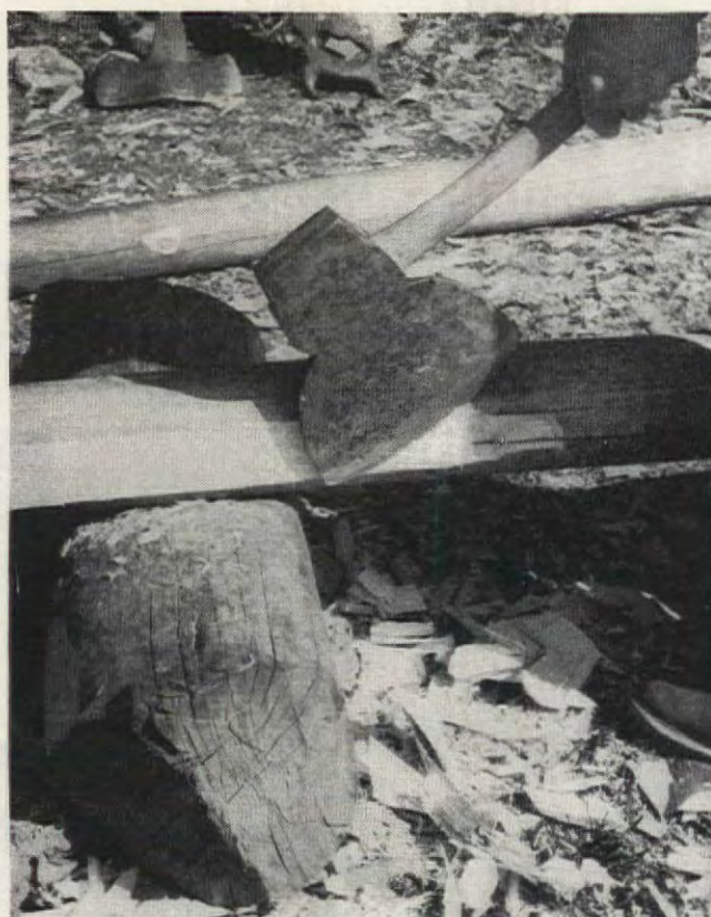
Top side of rafters is squared by hewing with a broad axe. Ceiling boards are laid on the flat surface. 2" x 2" strips on the ceiling above the rafters leave air space under roof boards
