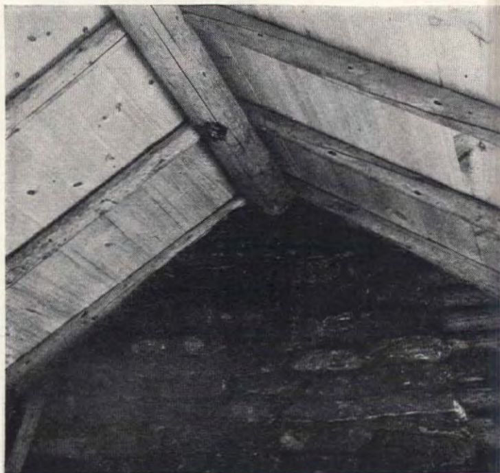
Above the native pine ceiling is 2" air space, spruce roof boards, roof felt, and slate
