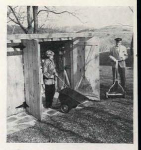
Simply constructed of 3/4 in. sheathing on a frame of 2 x 4's (which are doubled at the corners but single elsewhere) it combines a good appearance, efficiency, and tool care economy
