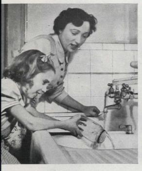
METAL EXPANDS when heated. Cover won't unscrew? Pour hot water over it and try again
