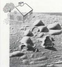
A too-thick coat of paint or cold and damp weather can be the cause of this wrinkling and sagging, even with a quality paint
