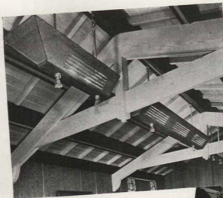
Slits in the improvised wood lighting troughs send a warm glow over painted beams, Modern fireplace and redwood walls in the living room
