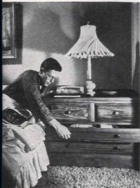
Passage between bedroom and bath identical sliding-door wardrobes in at either side, drawers for clothing. Luggage goes up top. Bed headboard, two 4-drawer units, frame for box-spring are all one continuous built-in unit
