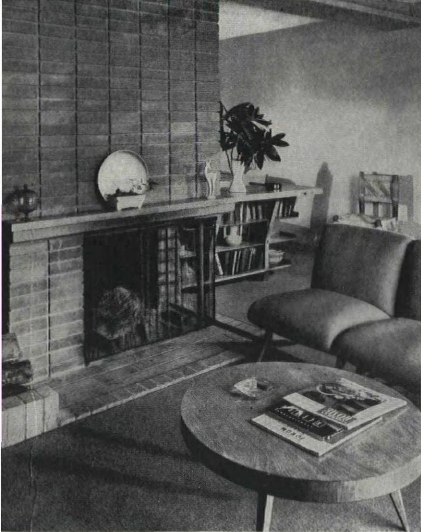
● Corner fireplace serves both living and dining rooms and has breast of concrete brick set with prominent vertical joints, blond wood mantel shelf blends naturally into built-in bookcase
