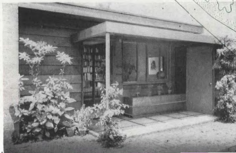
Ralph Clifford's own one-room house follows exterior pattern of his parents', with redwood siding; trim is deep gray-green instead of white. Covered porch has useful storage chest for garden tools and full view of attractive living room through the oversized windows
