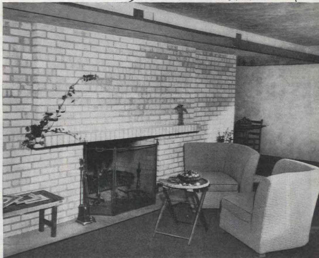
Indirect-lighting trough over living-room fireplace continues to the end of room to create difference in ceiling height at dining area
