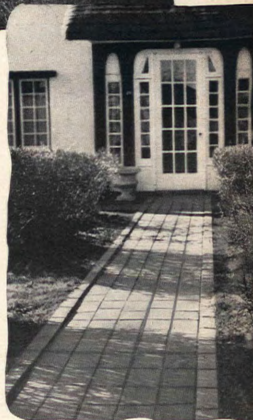
A cemented walk of tile or larger- than-ordinary brick, with neat raised border of same brick on edge
