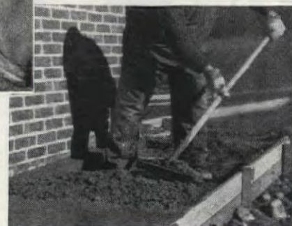
Concrete for making a walk is easily mixed in, then poured from a wheelbarrow
