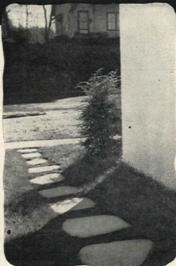
Simplest of all built paths—stepping-stones laid directly on firm earth
