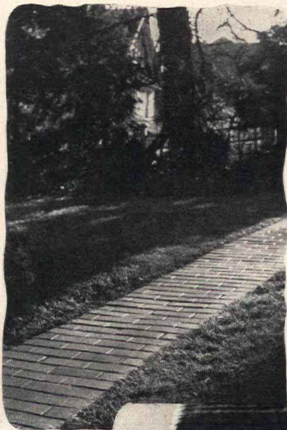
Hard brick laid flat on concrete and lower than grass to make mowing easier
