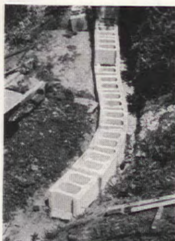
The retaining wall at an early stage showing brick construction and the "sweet curve" laid out with a hose
