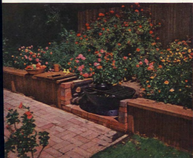
Grading left the patio 2 feet below surrounding level, so a retaining wall of railroad ties faced with redwood stakes was built as shown in plan. One-foot plank top is both seat and handy bench for preparing and serving food beside portable iron charcoal burner for which space was left in the wall
