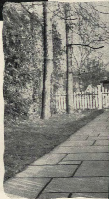
More formal effect—flagstone cut to sketch, laid without foundation or cement
