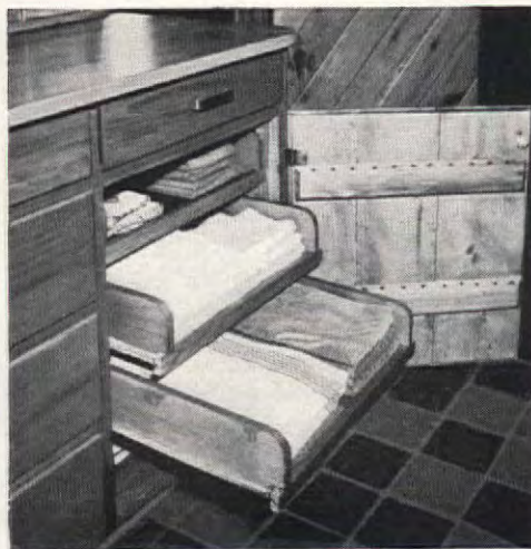
Every inch of space is utilized by converting cabinet to drawers. These three drawers pull out easily to almost the full 25-inch depth
