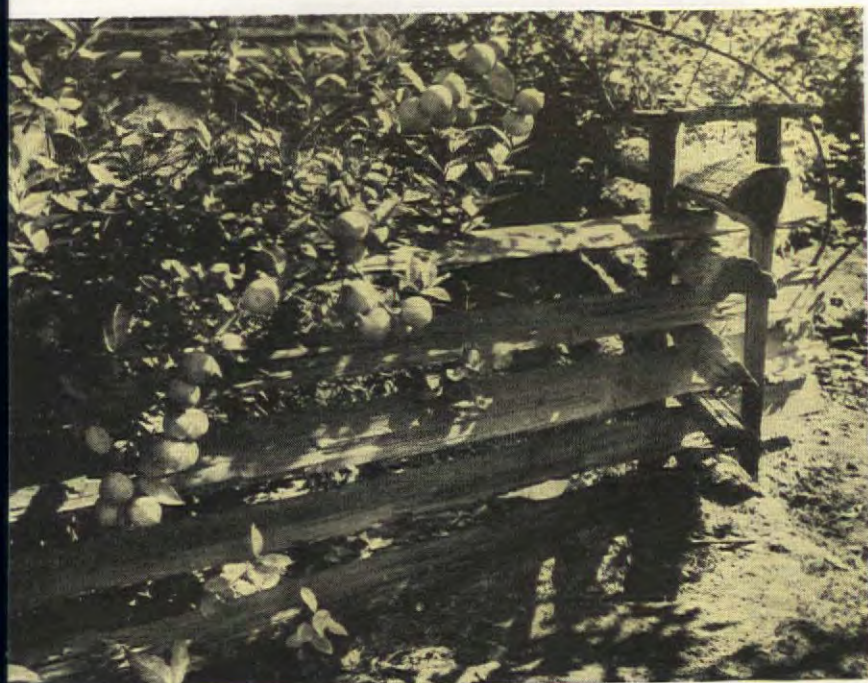
5. Old-time snake, or zig-zag, rail fence takes considerable space, but is picturesque, easy to make, secure, lasting
