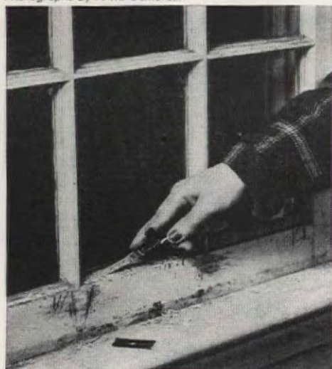
6. Now prepare wooden muntins. Scrape all mold and loose paint, especially in corners. Brush off with stiff wire brush so that surface is left smooth and clean
