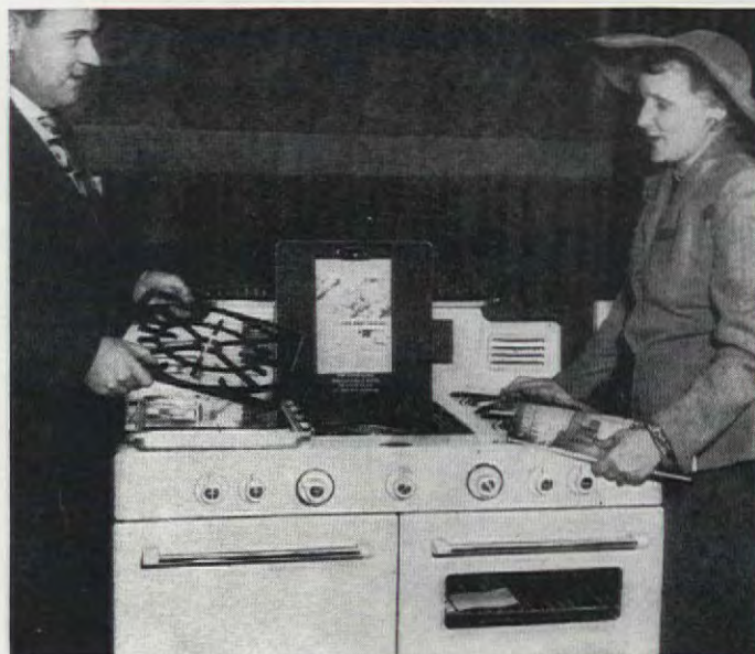
Sterling Beck of Estate explains extra-large griddle and foot-square replaceable grate to Editor Ramsay. With Grid-All, foods are grilled rather than fried, can be replaced by grate which holds jumbo kettles up to 21 qts.
