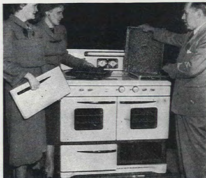
Julius Klein of Caloric shows our editors how their porcelain-enamelled broiler is designed so that not only broiler pan and rack, but entire broiler drawer and drawer front can be removed completely from range and washed in sink. To remove, lift latch on bottom of broiler. Is just as easy to replace
