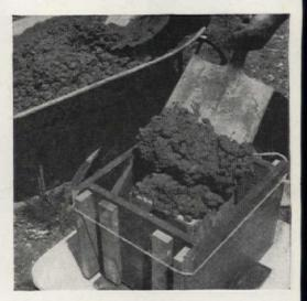
9 Shovel into space between molds but don't disturb them. Pack down so as to prevent voids; smooth surface with spade, trowel, or float. For smooth sides, work trowel inside forms
