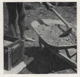
8 In metal wheelbarrow or mortar-box mix (dry) 6 shovels of washed gravel or broken stone, 6 of sharp sand, and 2 of cement. When well mixed, add water to give thick consistency
