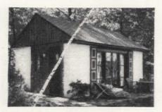
HOME STUDY PLAN NO. 12 One-room house 16 by 22 ft., waterproof cinder block painted on both sides, asbestos shingles. Kitchenette, closet, shower and lavatory. Built on concrete slab. Picture window 9 by 7 ft., glass doors
