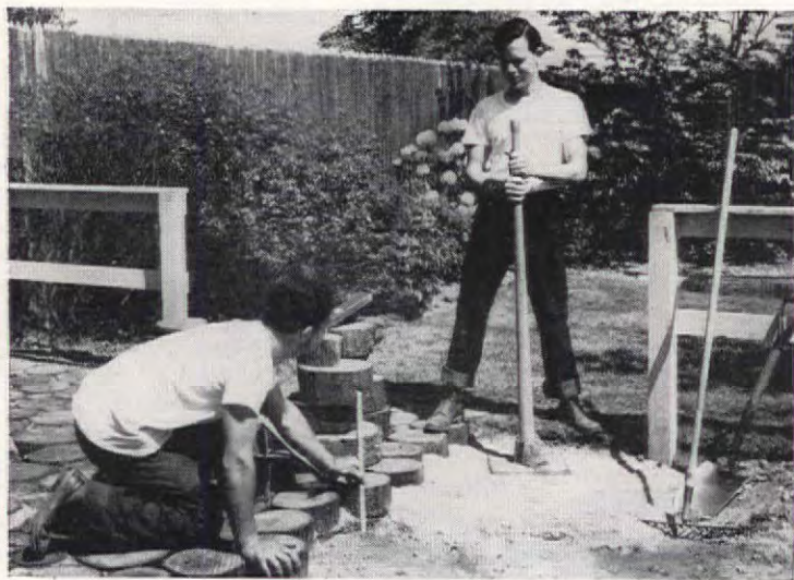
2. After gravel is raked level, tamped firm, spread on it at least 2 inches of clean builder's sand. Rake and tamp this level (as Don is doing). At left, Nicholas Gozo is showing, with ruler, depth of sand layer and of 5-inch log surfacing
