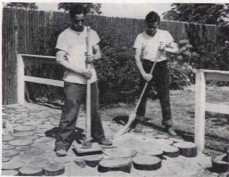
4. As soon as a few square feet are completed, tamp rounds to a smooth, permanent level. Immediately spread sand on top and sweep it back and forth until it fills all spaces completely. (Sand is better than soil and plants, which promote rotting.)
