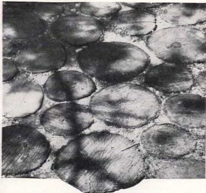
This student-made paving of oak and locust "rounds" at Farmingdale, Long Island, after 18 months is sound, firm, attractive. Durable wood and perfect drainage are essential
