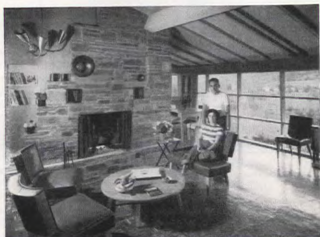
Fireplace is pride and joy of owners. Steel unit was used as form, covered with bluestone. Hearth 16 inches above floor, visible to all, eliminates bending down
