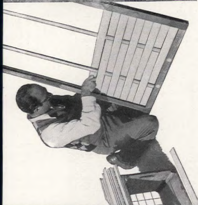
13. Inserting slats into frame is simple. Start from bottom, put one end in slot of frame, weave over one dowel, under other (alternate on every slat). Slip other end of slat into slot on opposite frame
