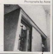
See how much a modern storage wall can help the looks as well as the usefulness of old houses. This capacious beauty, built of 5%-in. fir plywood, freed the old coat closet, which became a much-needed downstairs washroom. Storage wall is 2 ft. deep, reaches from floor to ceiling. It was pickled gray to match wallpaper. Other wood is same shade
