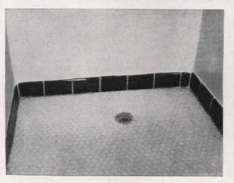
This is the finish! Gleaming enamel that makes a sparkling and thoroughly waterproof coating. It covers the patches at the base joining of the plaster and tile, and overlays the tile enough to prevent water leaks and cracks at this critical point. Showers are really a pleasure again!
