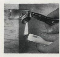
Thaw that frozen lock with dry heat, such as a candle flame, or electric soldering iron. Don't use hot water -it will rust lock, might refreeze
