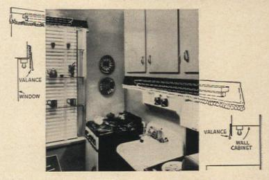
Lighten your "K.P." with well-illuminated working areas. Here fluorescent fixture is centered along the underside of the cabinet and concealed by a decorated plywood strip. Window valance also nests a good light
