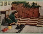
STEP 2... She puts tiles down in place, one at a time. When half the floor is covered, the adhesive is spread over the remaining half.
