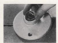
Shockproof empty sockets by inserting burned-out fuse. This will protect your curious small fry. The same trick will keep outdoor sockets in shape when not in use More on page 94
